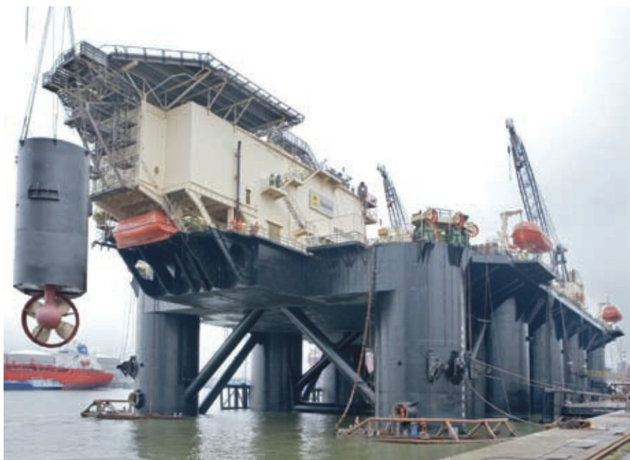
Keppel Verolme has finished installing one of the four thruster containers onboard Castoro Sei on time and safely
