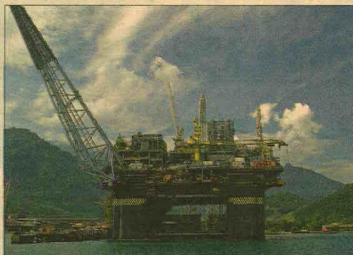
Track record: the P-52 semi-submersible in the final stages of commissioning at the BrasFels yard
